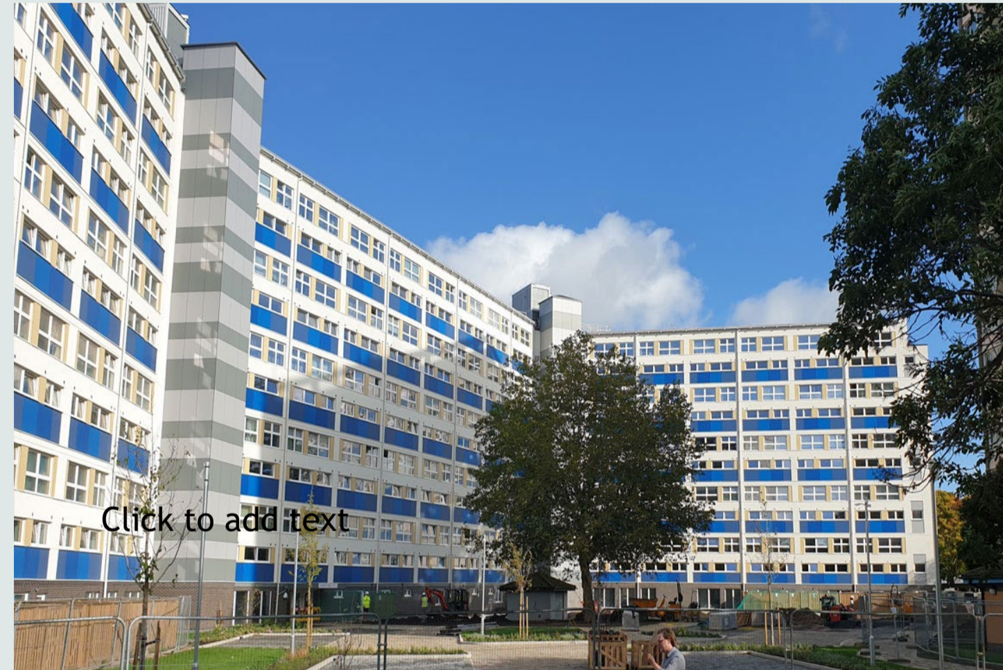
Wilmcote House Residential Refurbishment, Portsmouth ECD Architects
