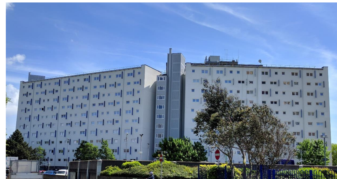
Wilmcote House Post-Retrofit
