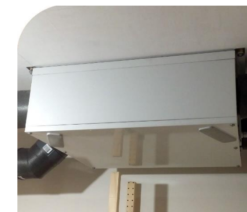
MVHR unit to be hidden above ceiling
