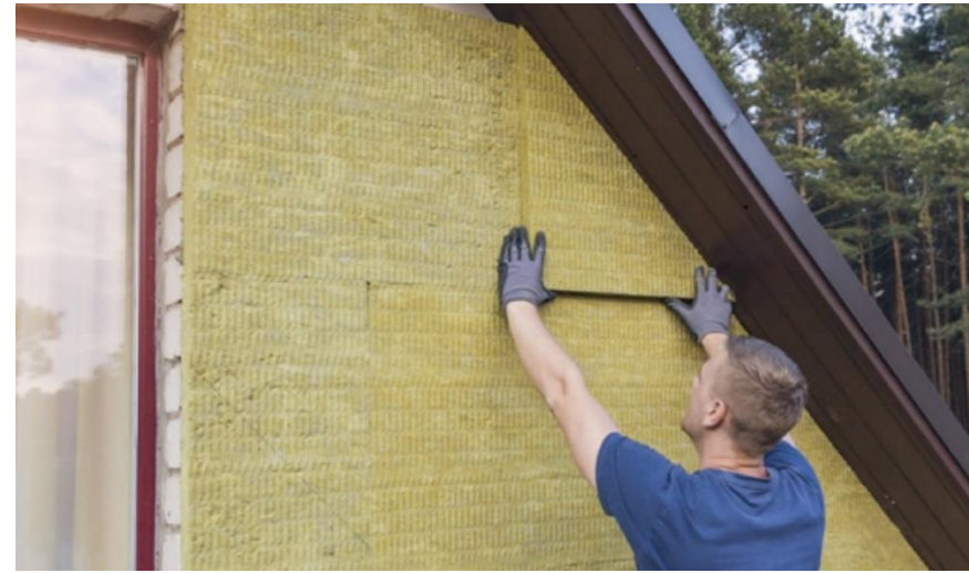
Adding external wall insulation to the outside of a building
