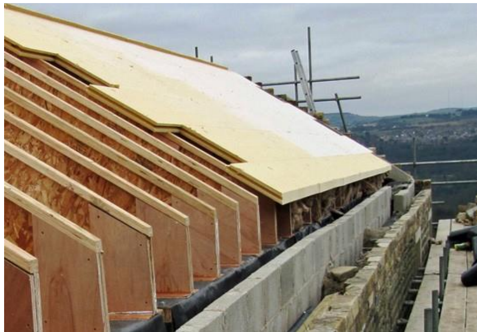
Insulation added between and over rafters
