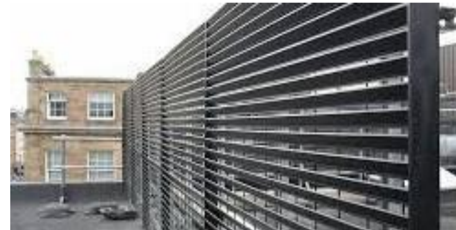
Example of screening of rooftop services
