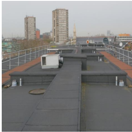
Existing roof (Typical build-up)
