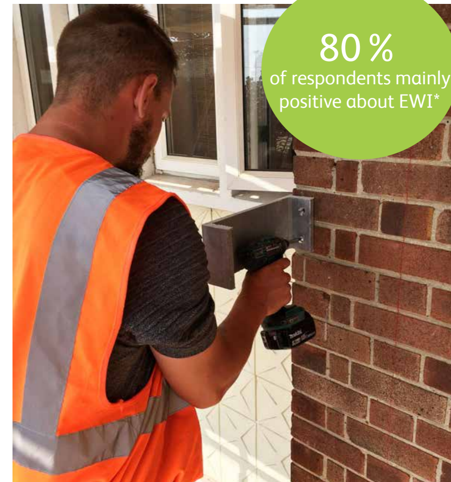
Figure 39 - EWI system construction process
