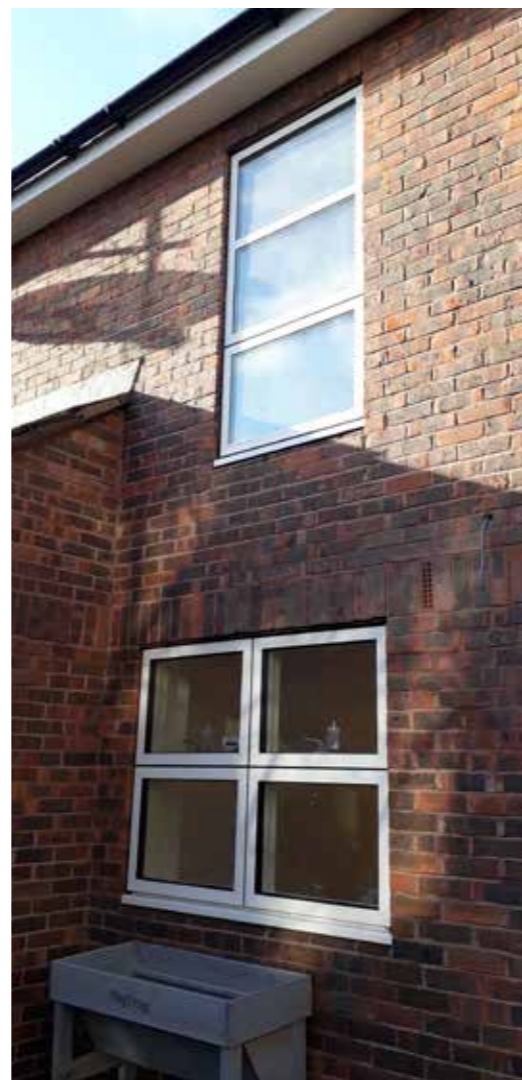
Figure 48 - New triple glazed windows at 50 Verity Close
