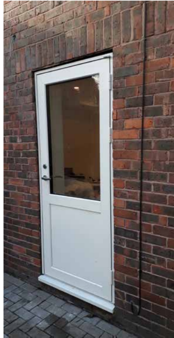
Figure 51 - New insulated triple glazed door at 50 Verity Close
