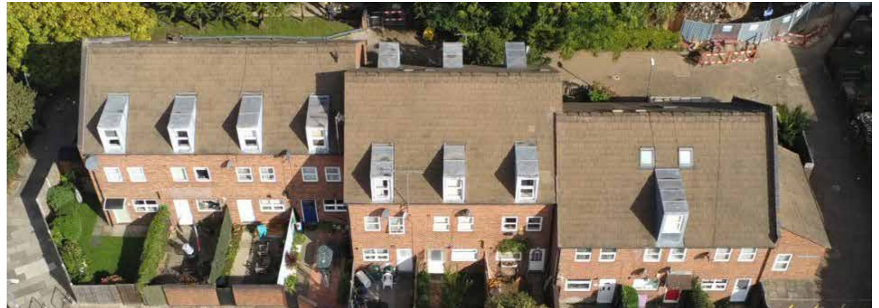
Figure 45 - Verity Close Roof View
