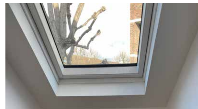
Figure 50 - New triple glazed roof-lights at 50 Verity Close. These examples are made by Velux, and can function like other Velux roof-lights
