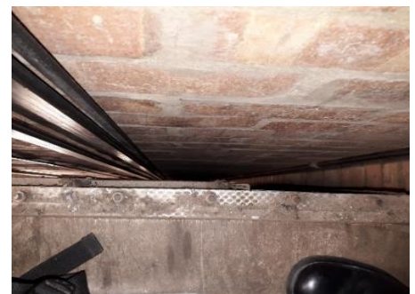
Rear of lift car to rear wall of shaft
