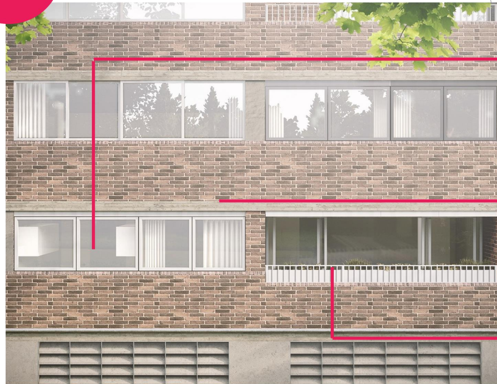
Image of exterior of external refurb pilot flat
