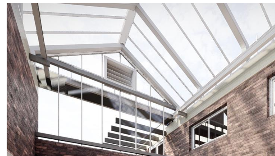
Automatic Opening Vents (AOVs), to be replaced in roof lights
