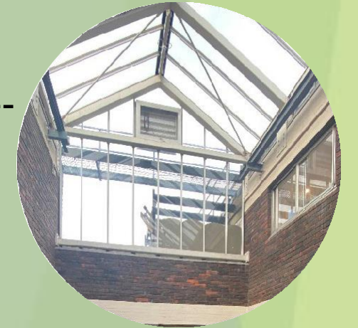
New rooflights to common areas with new smoke ventilation
