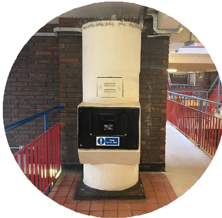
Existing internal bin chutes
