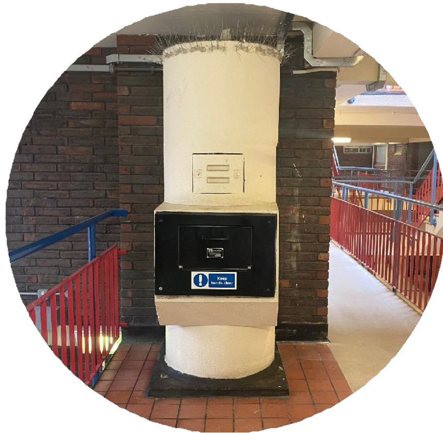
Existing internal bin chutes
