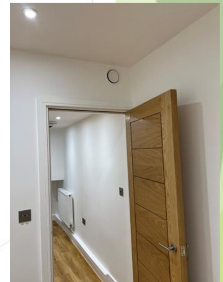
MVHR plastic ductwork
