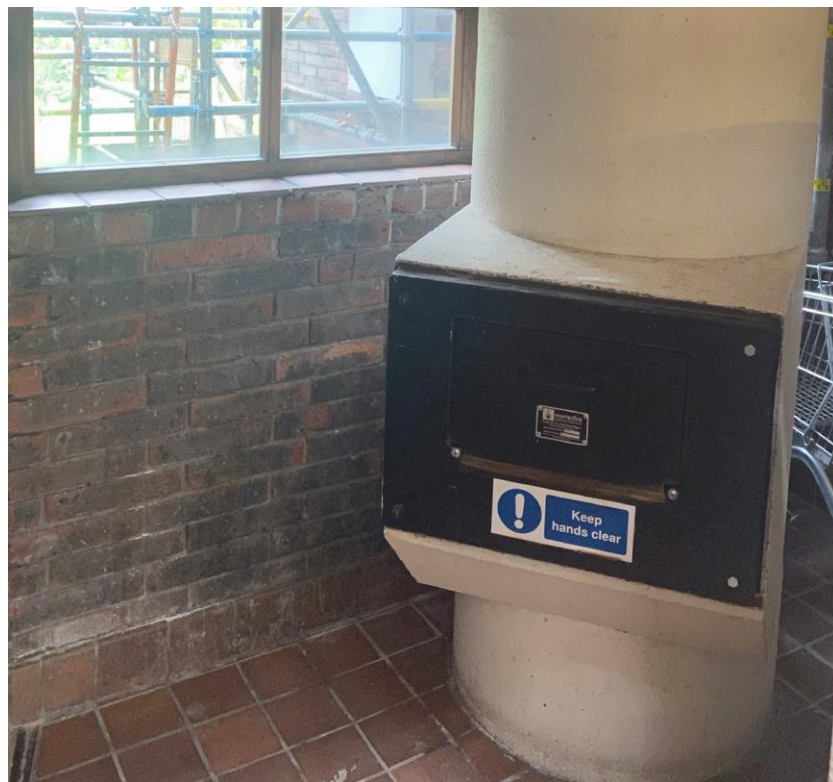
Existing bin chutes
