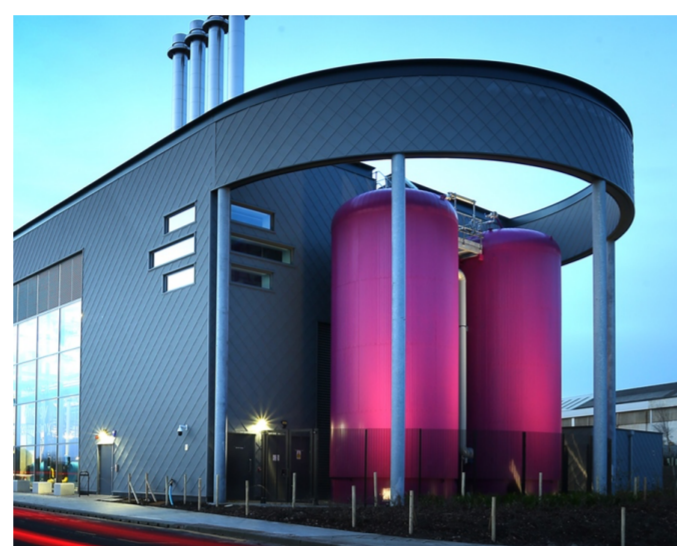
Example 2: Part of building A water store becomes part of the building.
