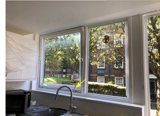
Completed refurbishments With kitchens by windows.
