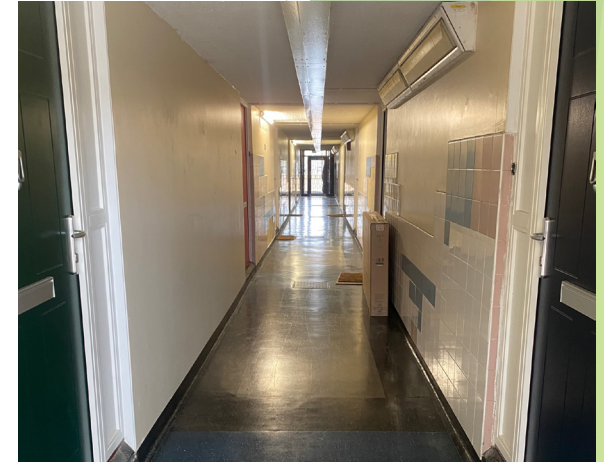
Existing condition - Upper Talbot Walk
