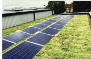
BRAMLEY HOUSE: EXAMPLE OF PROPOSED ROOF
