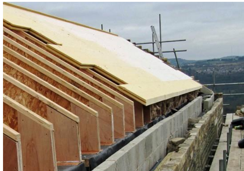
Insulation added over rafters
