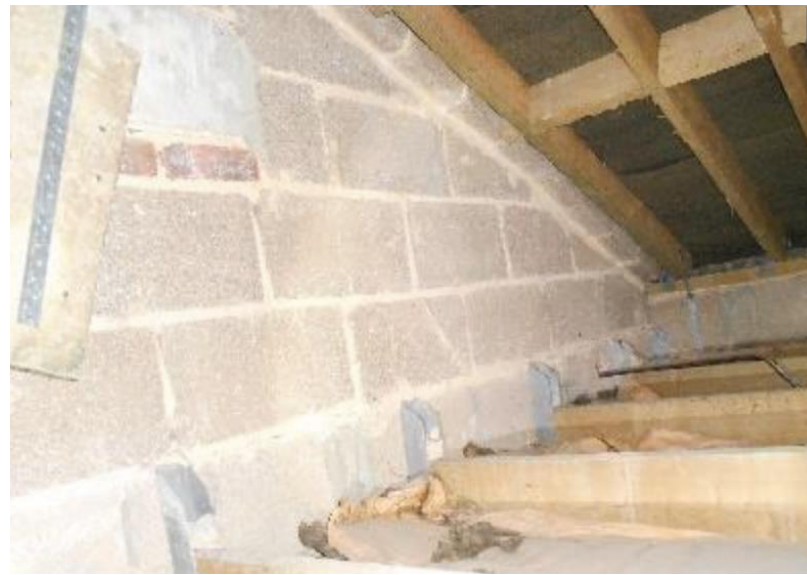
Existent roof space
