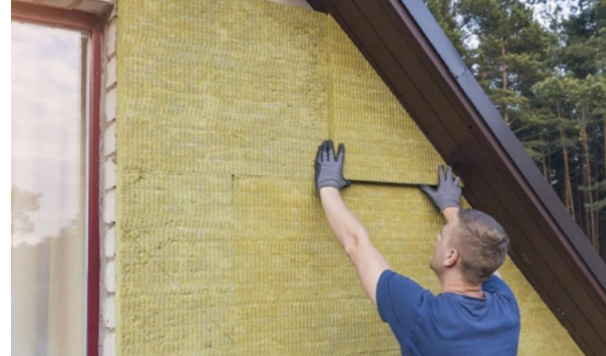
Adding external wall insulation to the outside of a building
