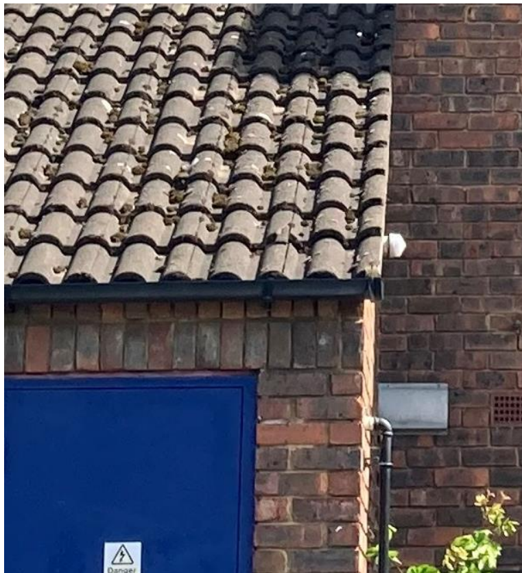
Existing roof tiles
