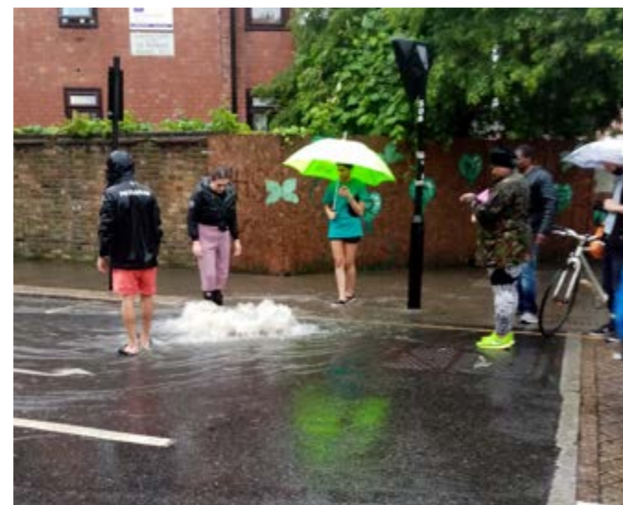
Overflowing at the Thames Water manhole on St Marks Road (refer to point 1 above)
