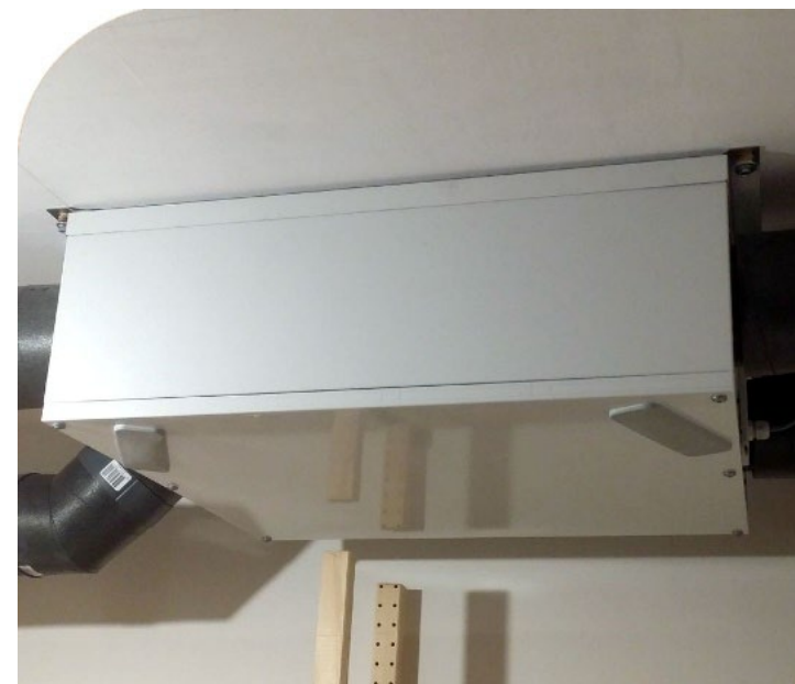
MVHR unit to be hidden above ceiling
