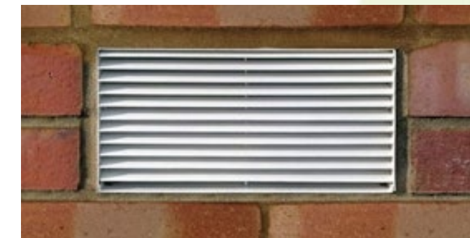
Example of MVHR vents on the outside of the home
