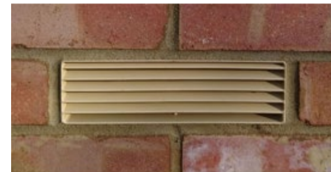
Example of MVHR vents on the outside of the home
