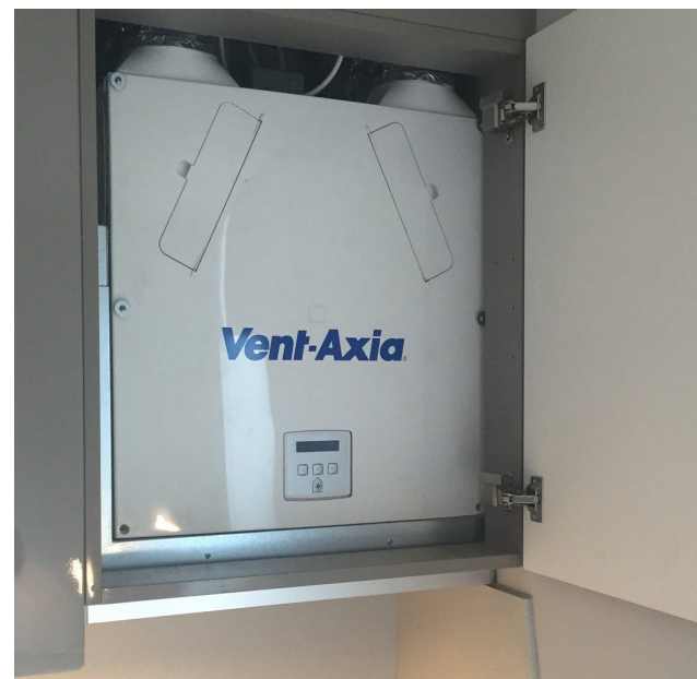
MVHR unit inside cupboard
