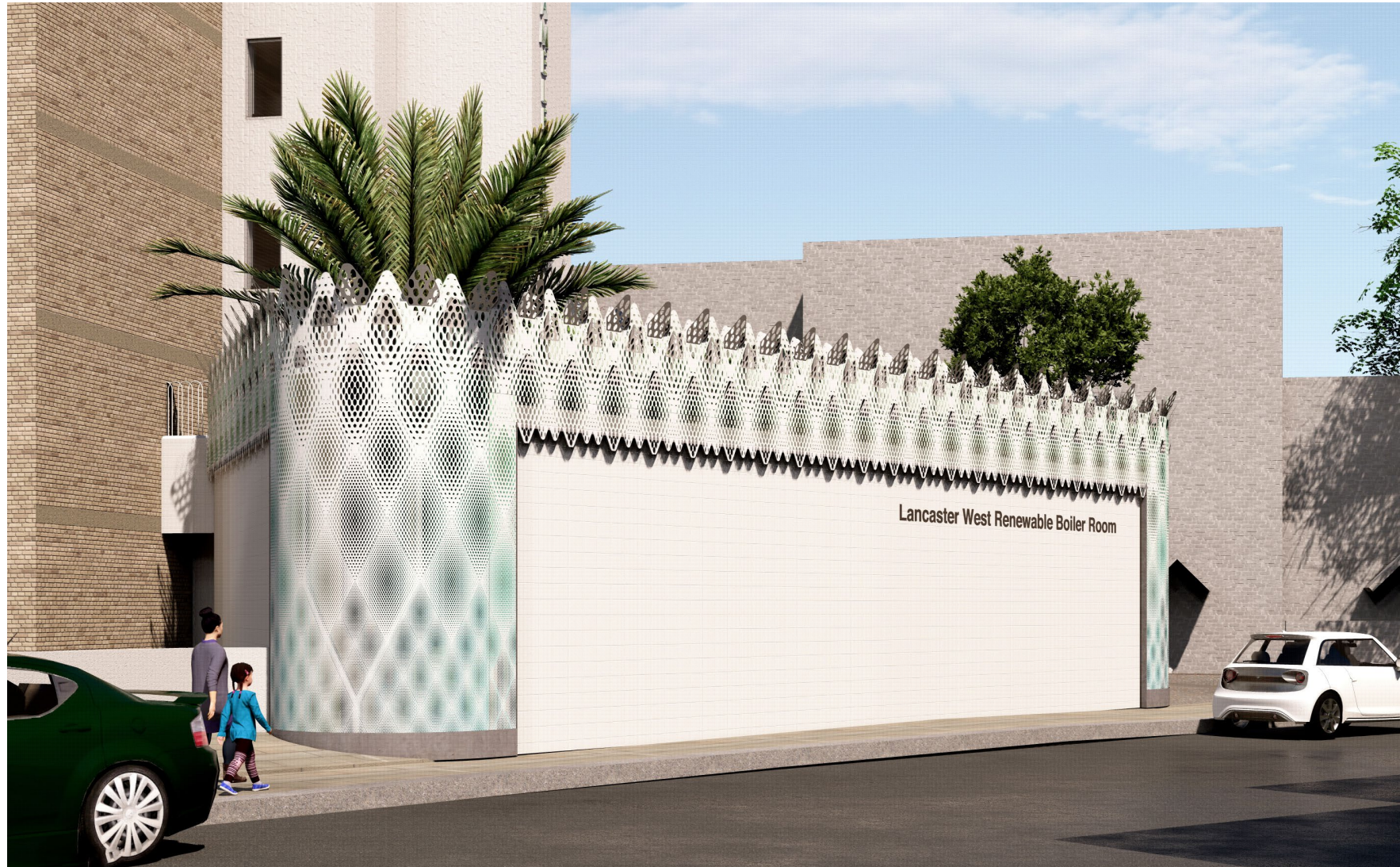
Energy plant on Clarendon Road near Safestore
