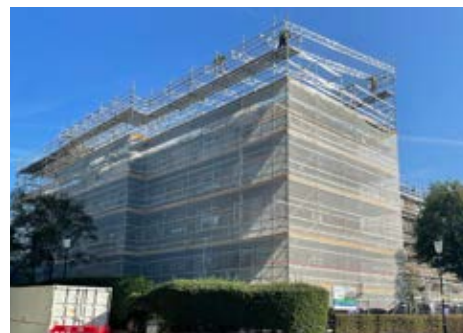
The carbon-neutral refurbishment works at Treadgold House are underway.
