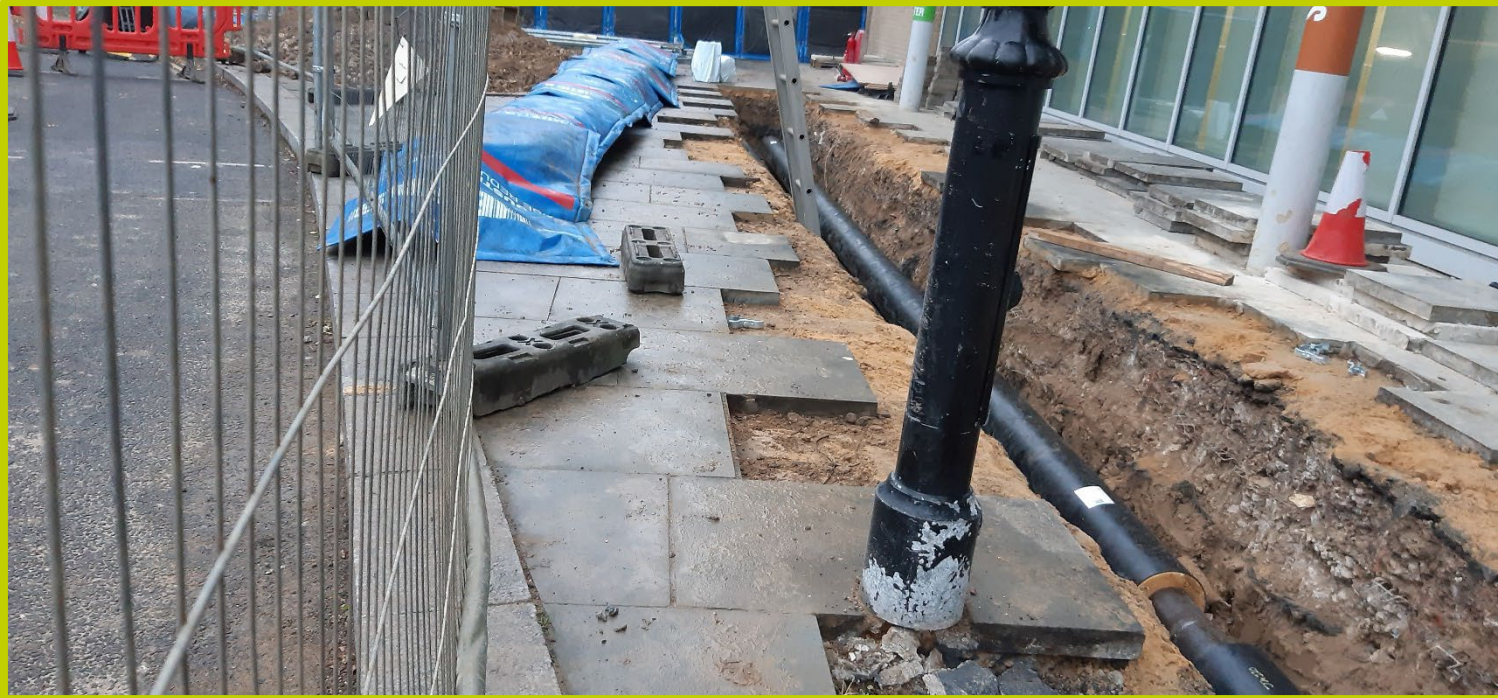
Bomore Road during works
