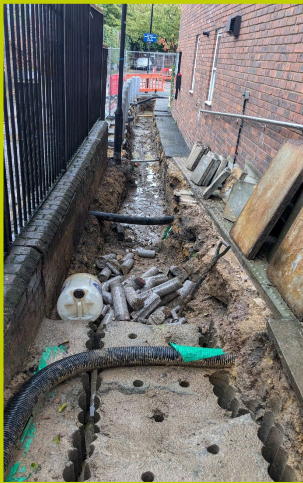
Cambourne Mews during works
