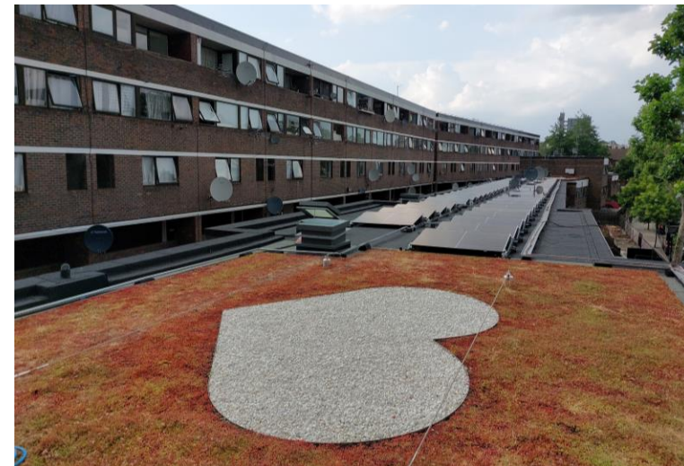
Image 3: picture of Camelford Court's bio-solar roof, with 98 Solar PV panels.
