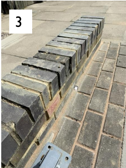
Brick work – requested to start again
