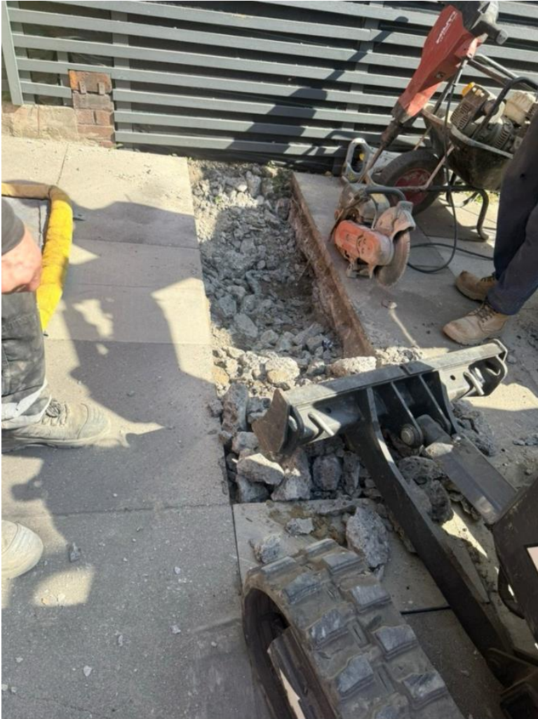
Ground conditions outside lower clarendon Note – concrete slab below pavers which lead to significant high impact works and increased programme
