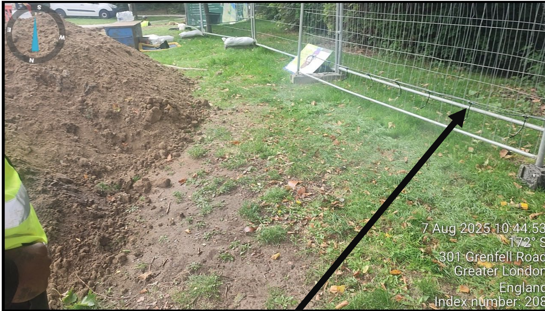
Dust suppression in full operation (mistlers are attached to fencing)
